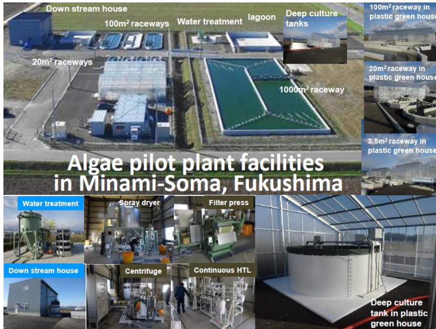
Figure 81. Algae pilot plant in Fukushima.
