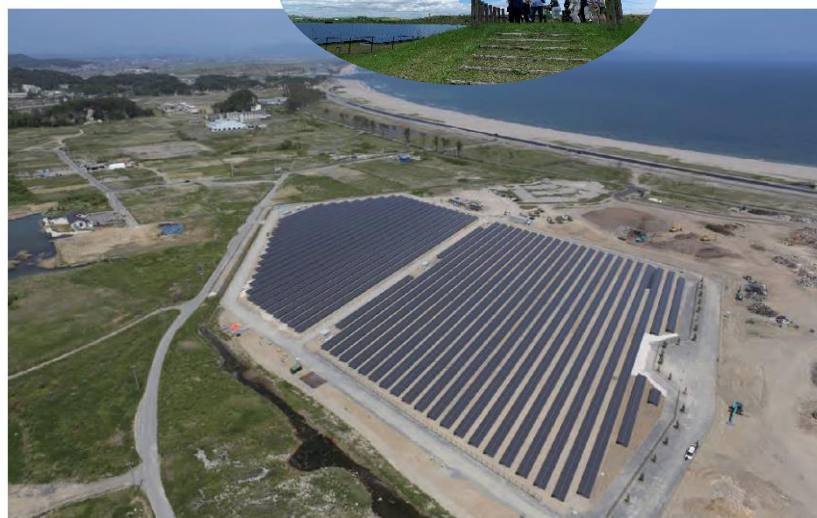
▲ Okumatsushima “Kizuna” solar park (sustainable economy and effective utilization of disaster stricken areas)
